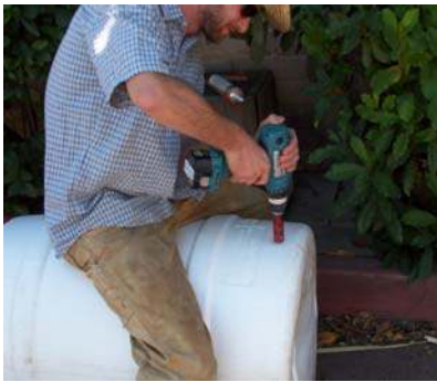
Step Three: Drill Holes in Barrels
