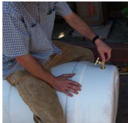
Step Four: Attach Bib Hose Connector and Valve
