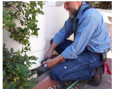
Step Five: Attach PVC to Barrels
