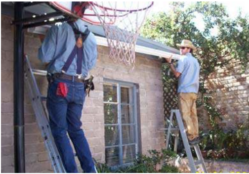
Step One: Install Gutters
