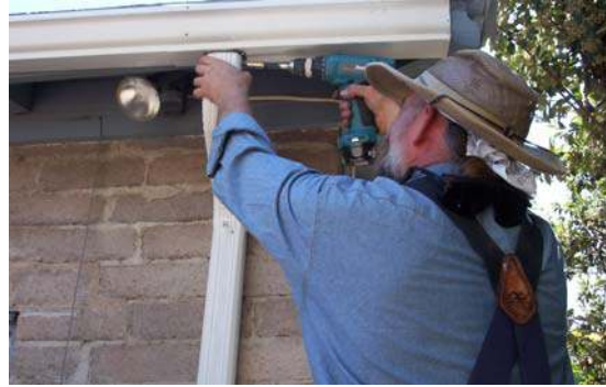
Step Two : Attach Downspouts
